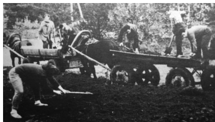
Horse-drawn carts were hired to carry out excavation work
