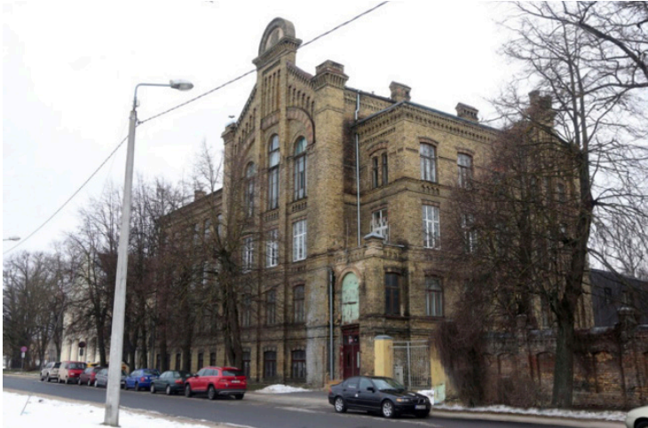
The building at 2 Abrenes Street in Riga—one of the focuses of restitution—was a Jewish vocational school in the 1920s and 1930s
