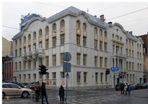
The building on 6 Skolas Street after renovation.
